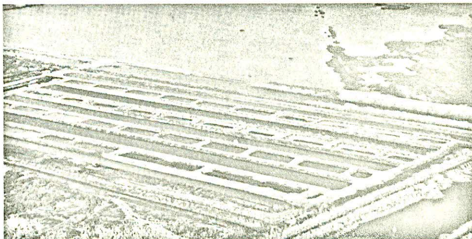
A total of 51 ponds have been constructed on the Rockefeller Wildlife Refuge for fishery studies. These ponds, ranging in size from 0.1 to 5.0 acres, are constructed in such a manner as to allow salt water collection from a tidal bayou leading to the Gulf of Mexico or fresh water from a canal draining the fresh water marshes. Marsh pond construction is unlike any other. Note the dragline on mats.
